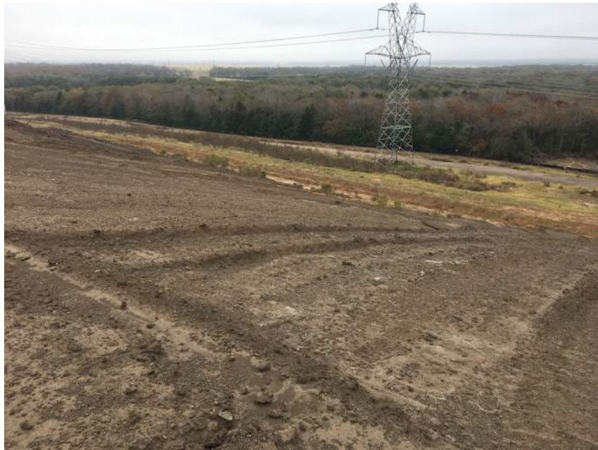
Photo No. 3 – South side slope, view southeast.
