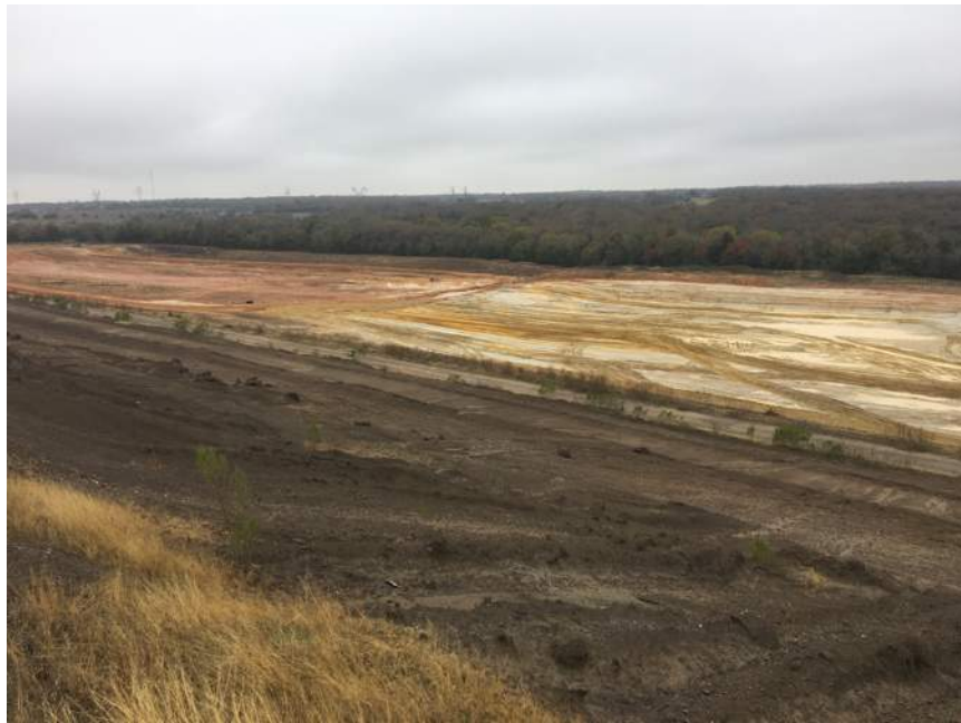
Photo No. 9 – North Side Slope, lateral expansion area, view northwest.
