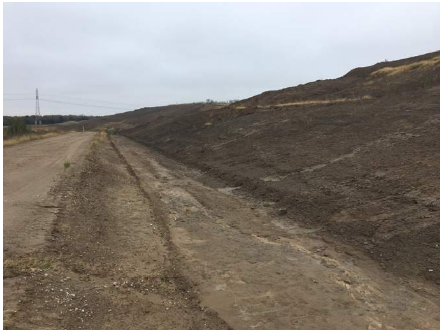
Photo No. 8 – East side slope, perimeter drainage ditch, view south.
