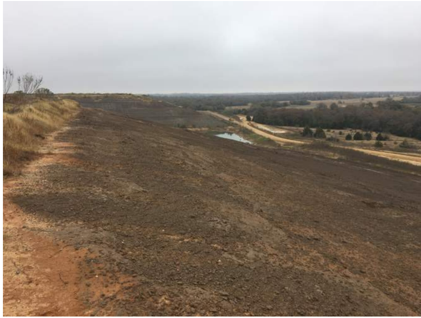
Photo No. 5 – East side slope, view north.
