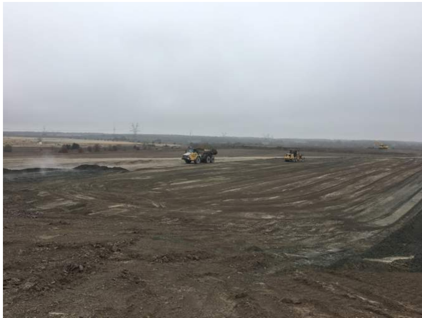
Photo No. 11 – Active disposal area, view northwest.
