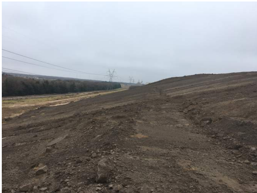
Photo No. 4 – South side slope, view west.
