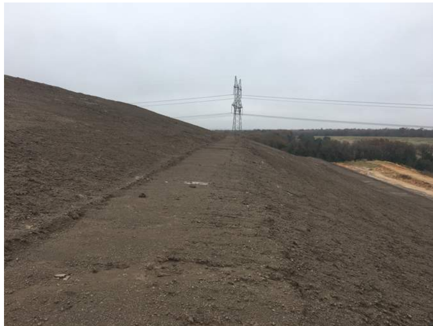
Photo No. 2 – West side slope (mid-slope), view south.
