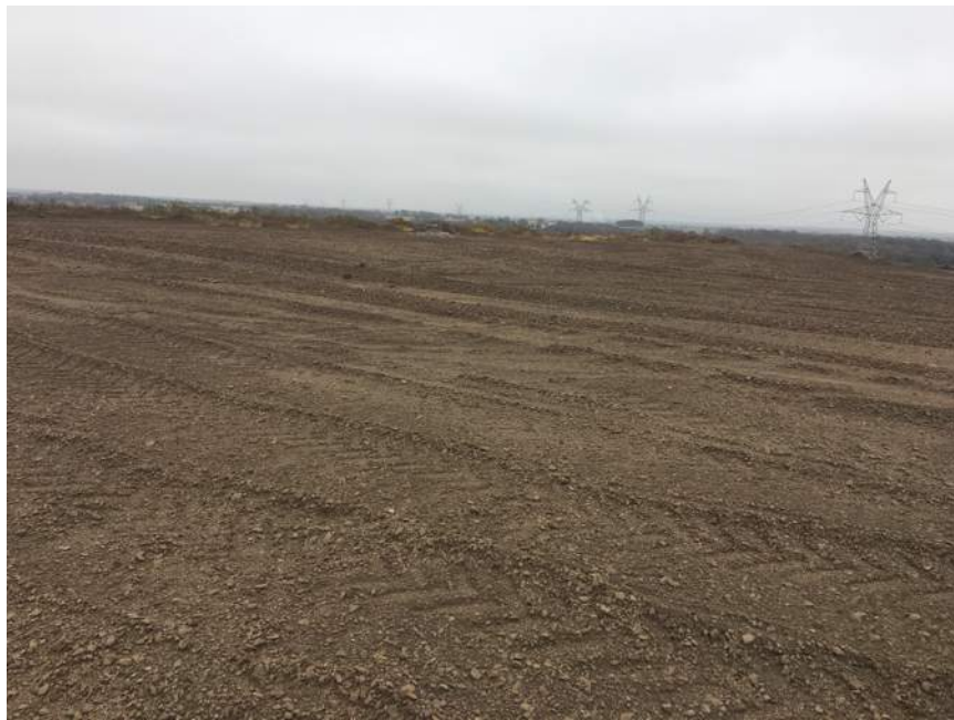
Photo No. 14 – Milled CCR for beneficial reuse, view east.
