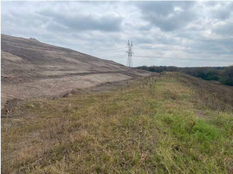
Photo No. 12 – West perimeter drainage ditch, view south.
