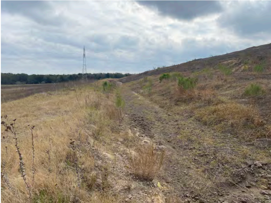
Photo No. 10 – East perimeter drainage ditch (south of Pond No. 3), view south.
