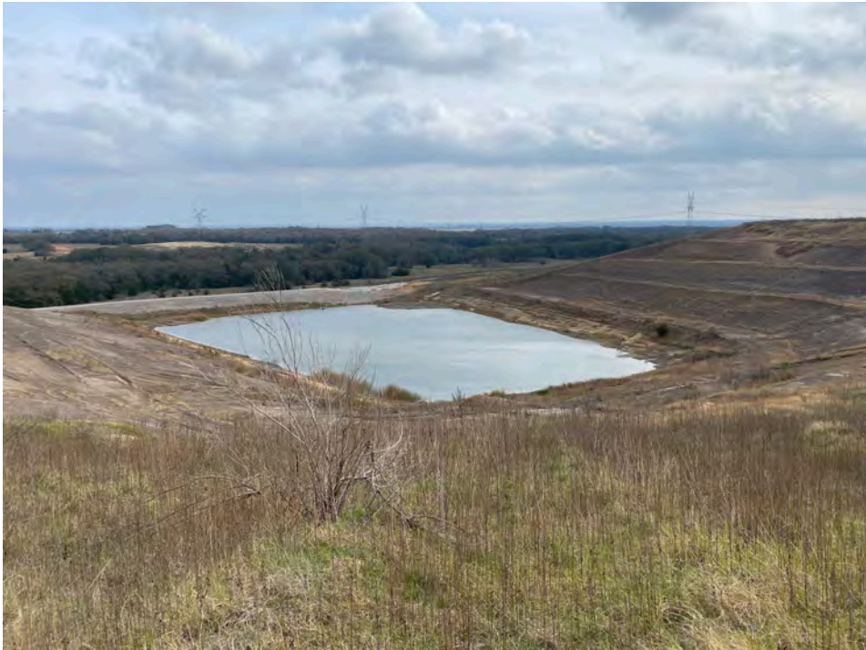
Photo No. 4 – Stormwater Pond No. 3, view southeast.
