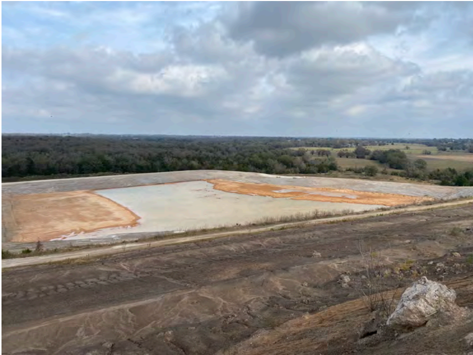
Photo No. 5 – Stormwater Pond 009, view northeast.
