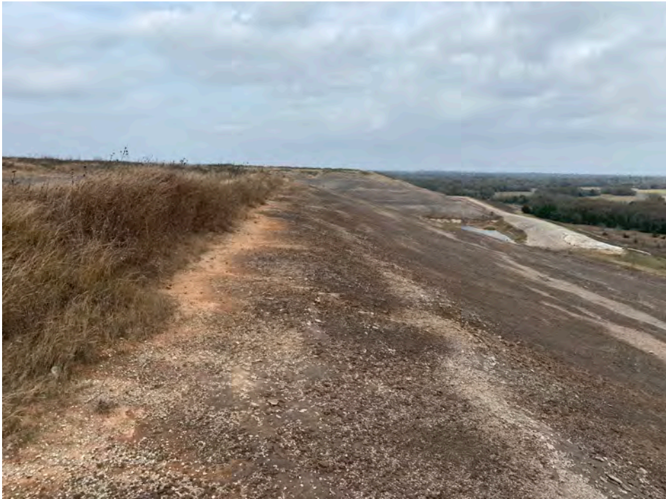
Photo No. 9 – East side slope crest, view north.
