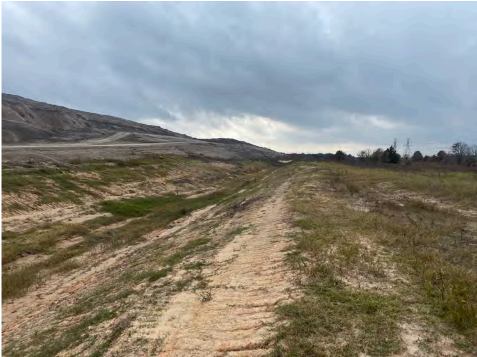
Photo No. 1 – North portion of west perimeter drainage ditch, view south.
