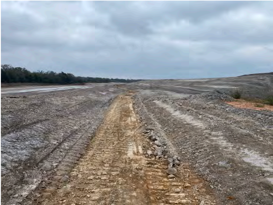
Photo No. 3 – North perimeter drainage ditch, view east.
