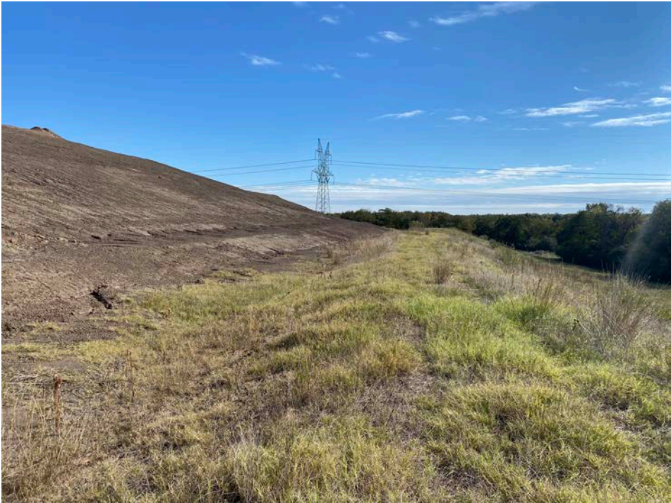
Photo No. 14 – West slope and west perimeter ditch, view south
