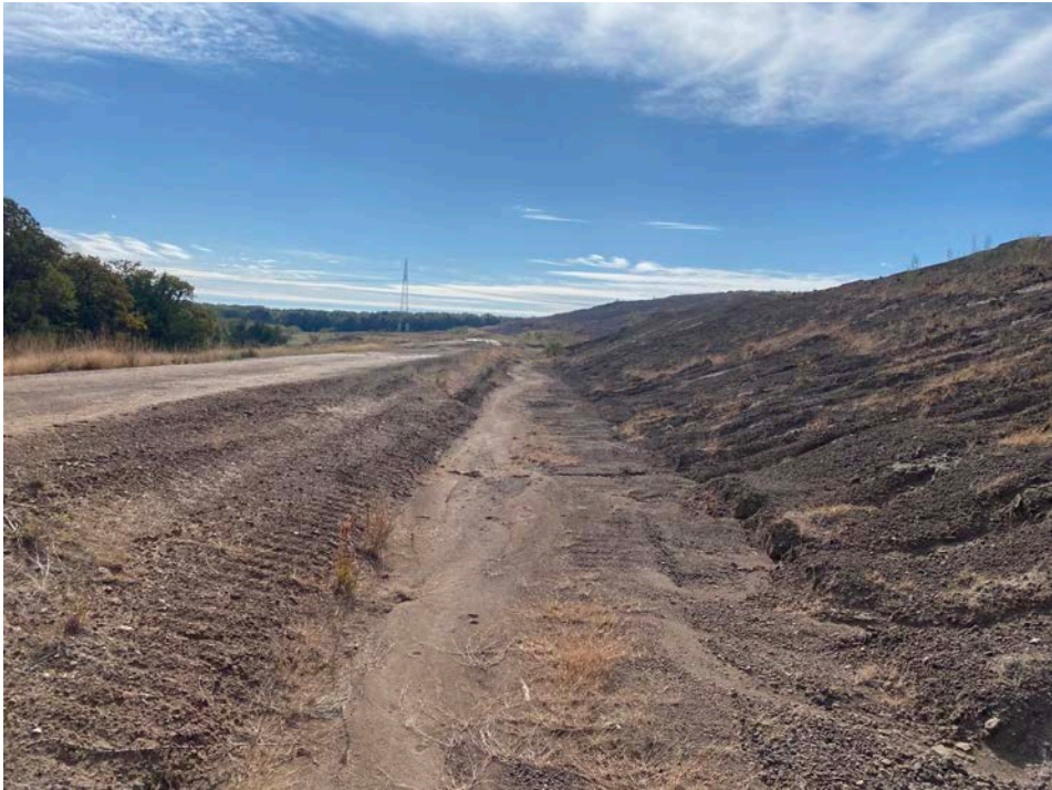
Photo No. 4 – East perimeter ditch, view south.
