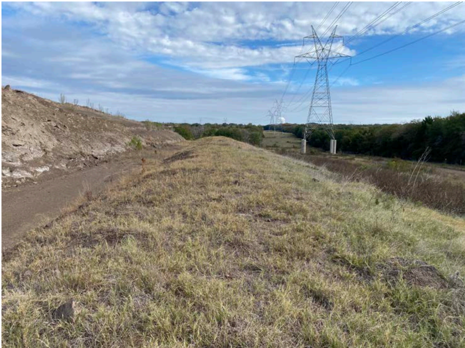
Photo No. 8 – South perimeter ditch, view east.
