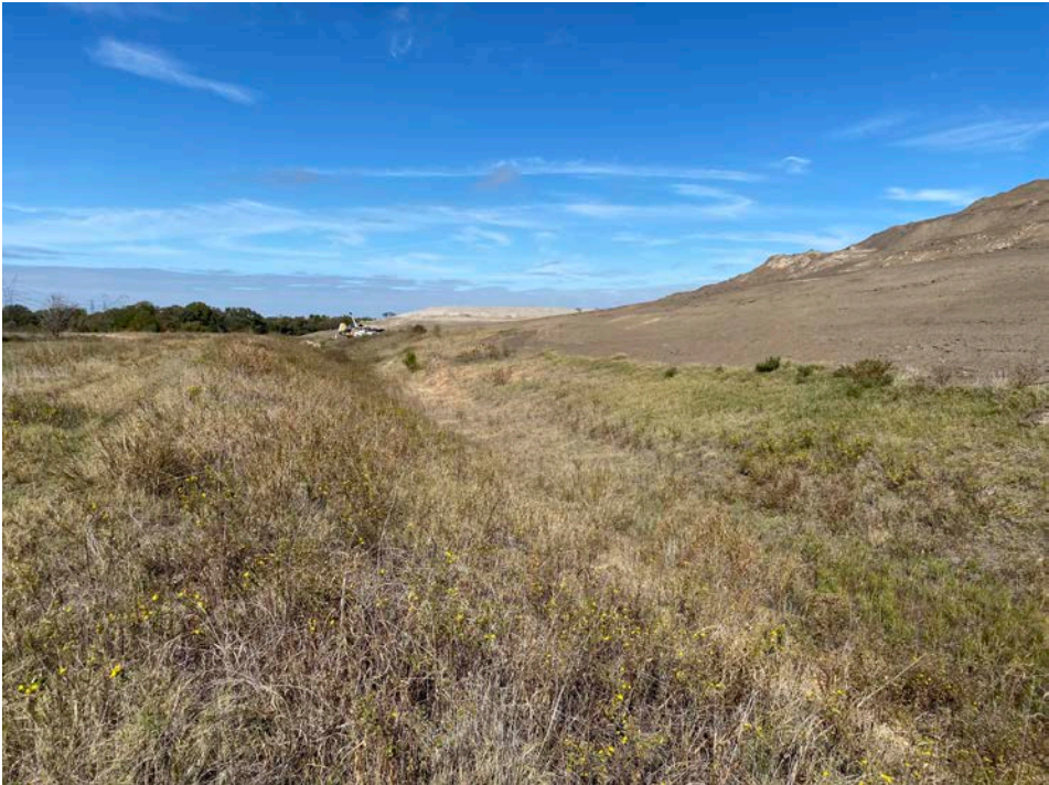
Photo No. 13 – West perimeter ditch, view north
