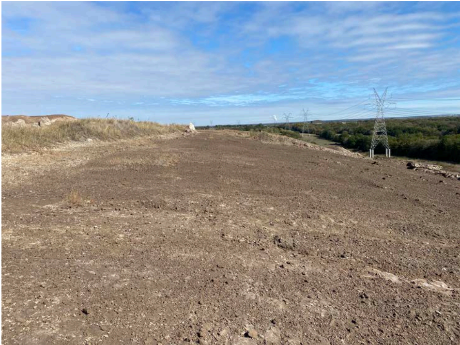
Photo No. 11 – South side slope crest, view east.
