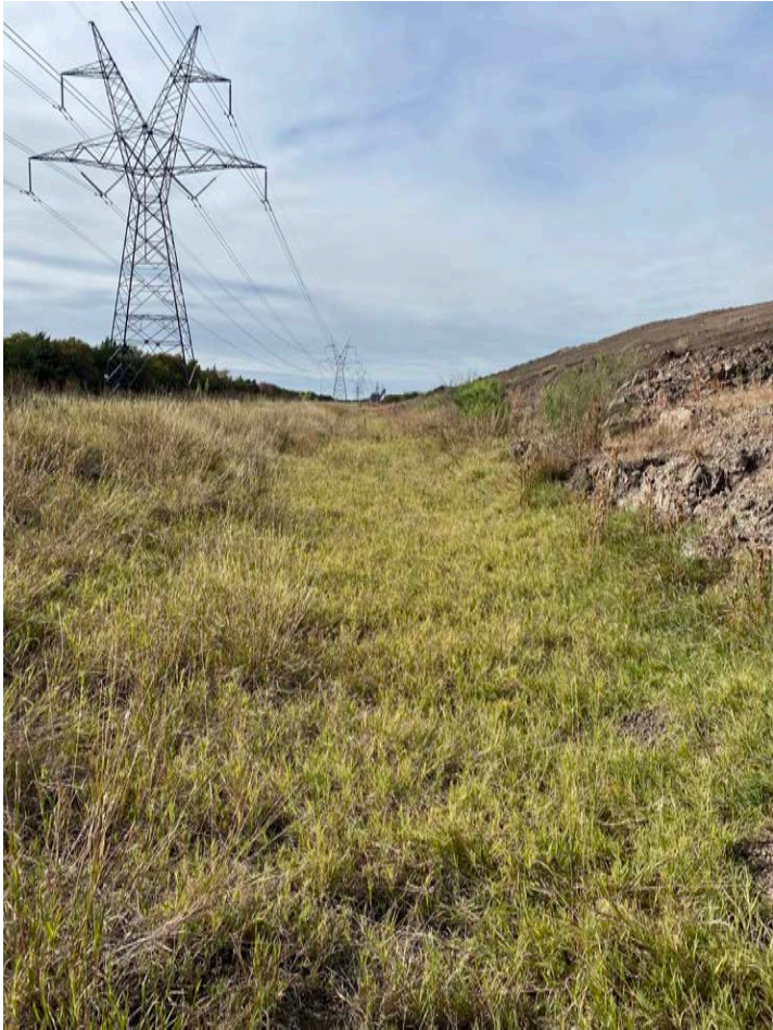
Photo No. 7 – South perimeter ditch, view west.
