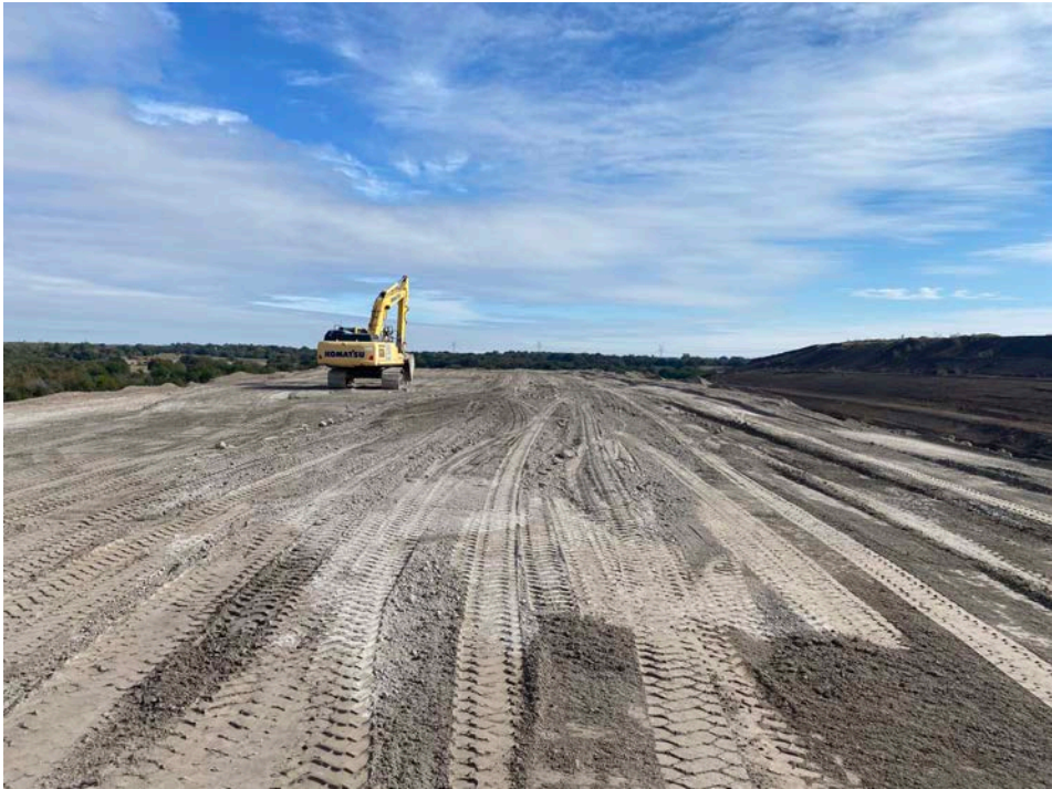
Photo No. 3 – Active disposal area, view east.
