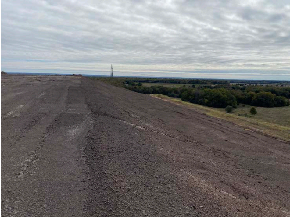
Photo No. 10 – West side slope, crest, view south.
