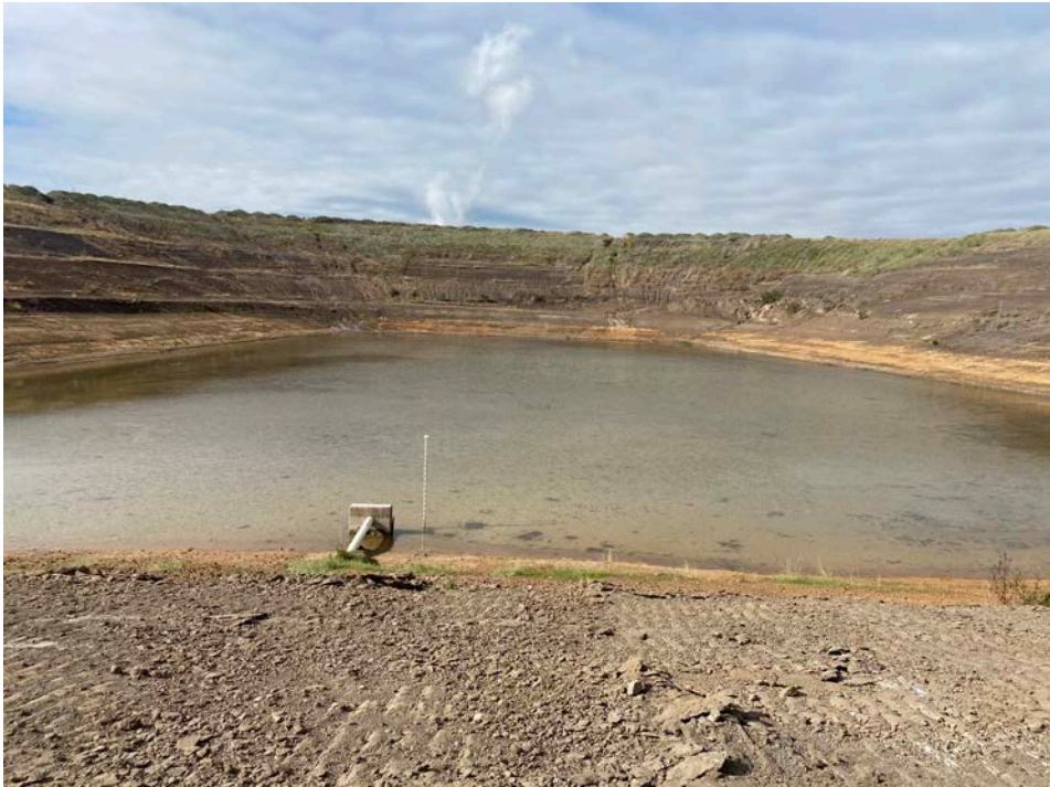
Photo No. 5 – Stormwater Pond 003, view west.
