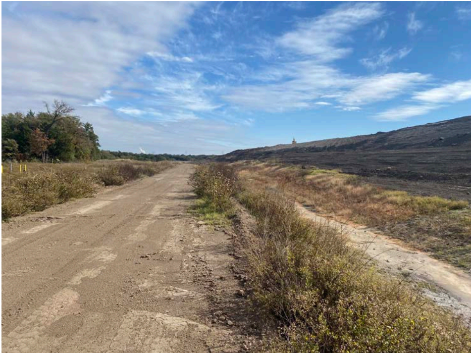
Photo No. 1 – North perimeter drainage ditch, view east.
