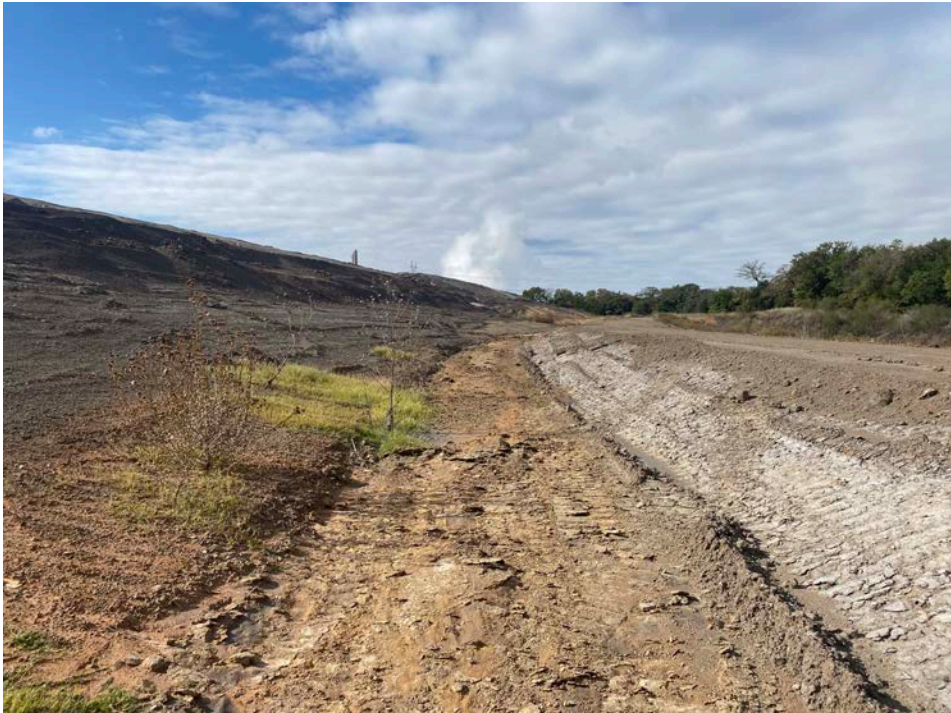
Photo No. 2 – North perimeter drainage ditch, view west.
