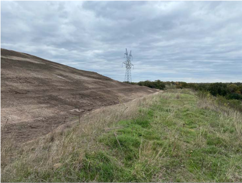
Photo No. 3 –West slope perimeter drainage ditch, view south.
