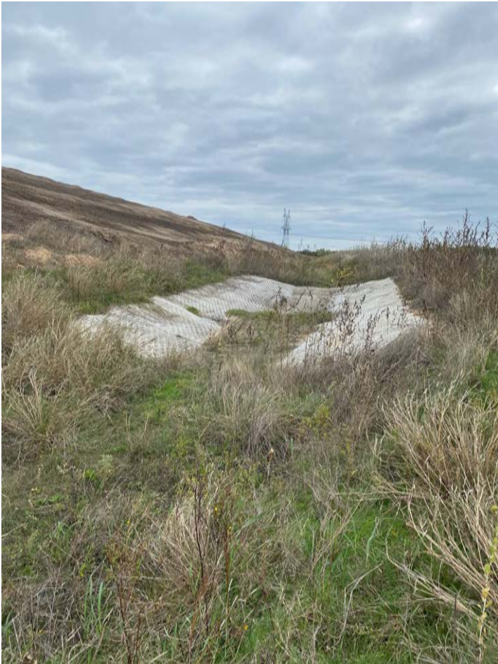
Photo No. 2 – West perimeter drainage ditch, drop structure, view south.
