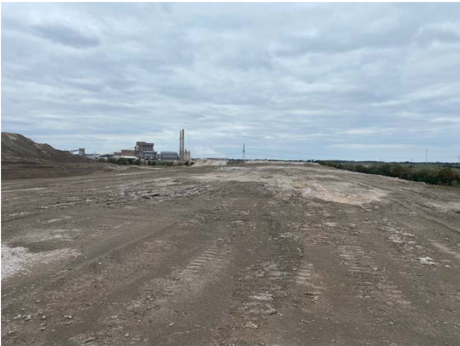
Photo No. 7 – Disposal Area North, view west.
