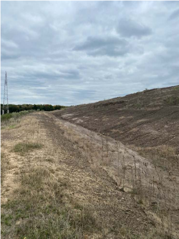
Photo No. 8 – East perimeter ditch, view south.
