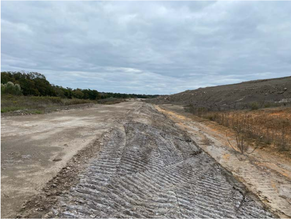
Photo No. 4 – North perimeter ditch, view east.
