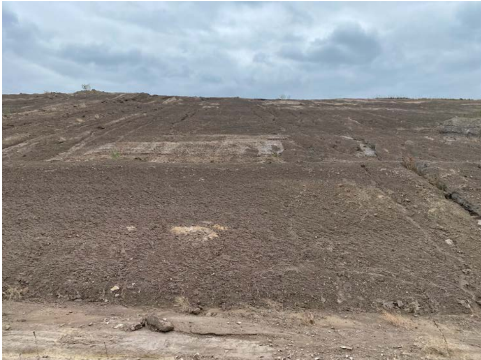
Photo No. 11 – South side slope (from toe), view north.
