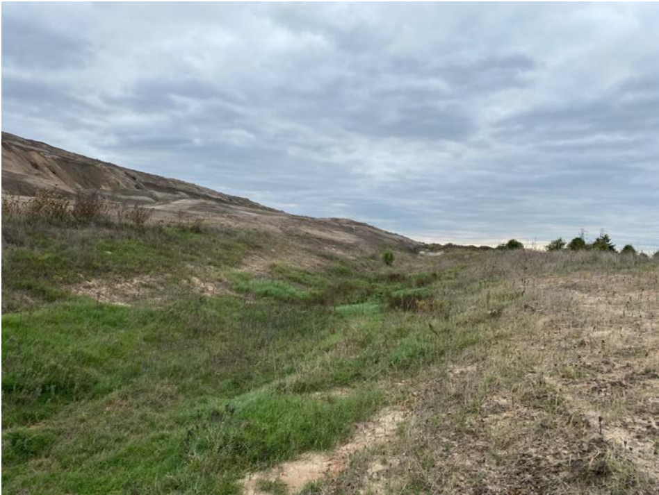
Photo No. 1 – West perimeter drainage ditch, view south.
