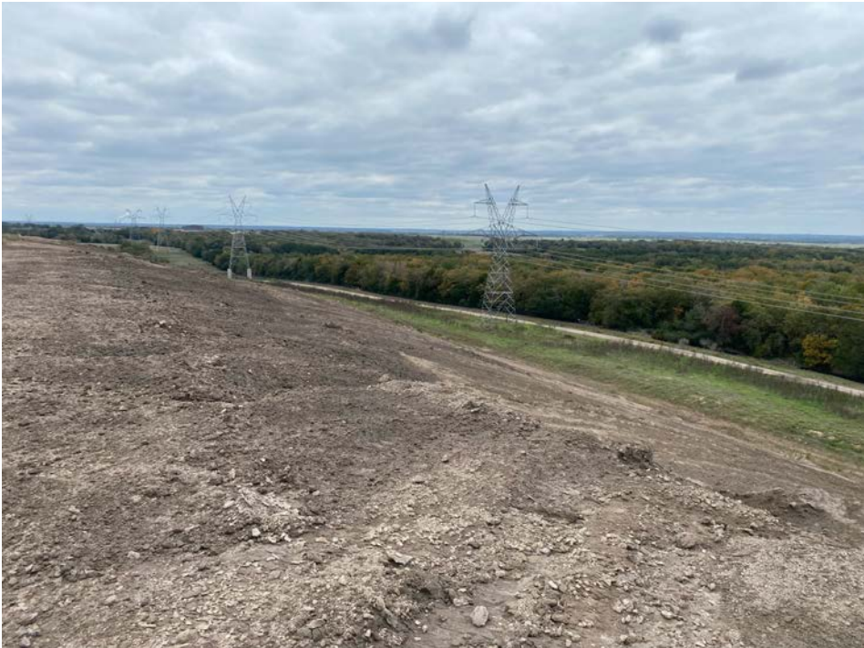
Photo No. 12 – South side slope (from crest), view southeast.
