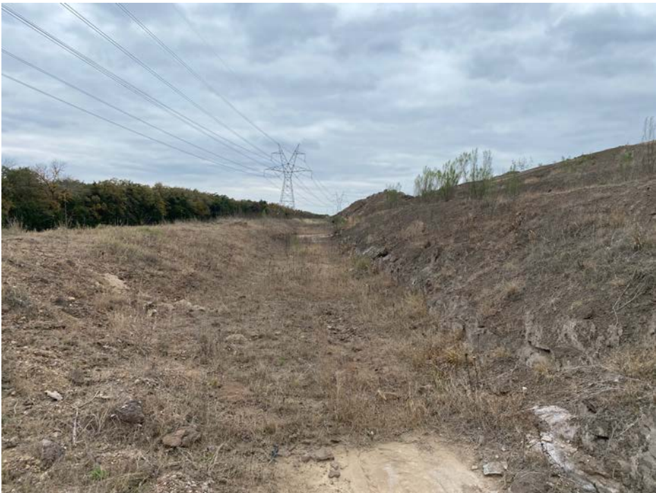
Photo No. 10 – South perimeter ditch, view west.
