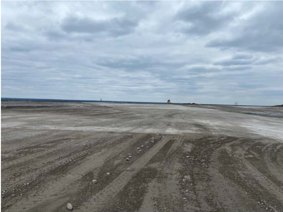
Photo No. 13 – Disposal Area South, view south.
