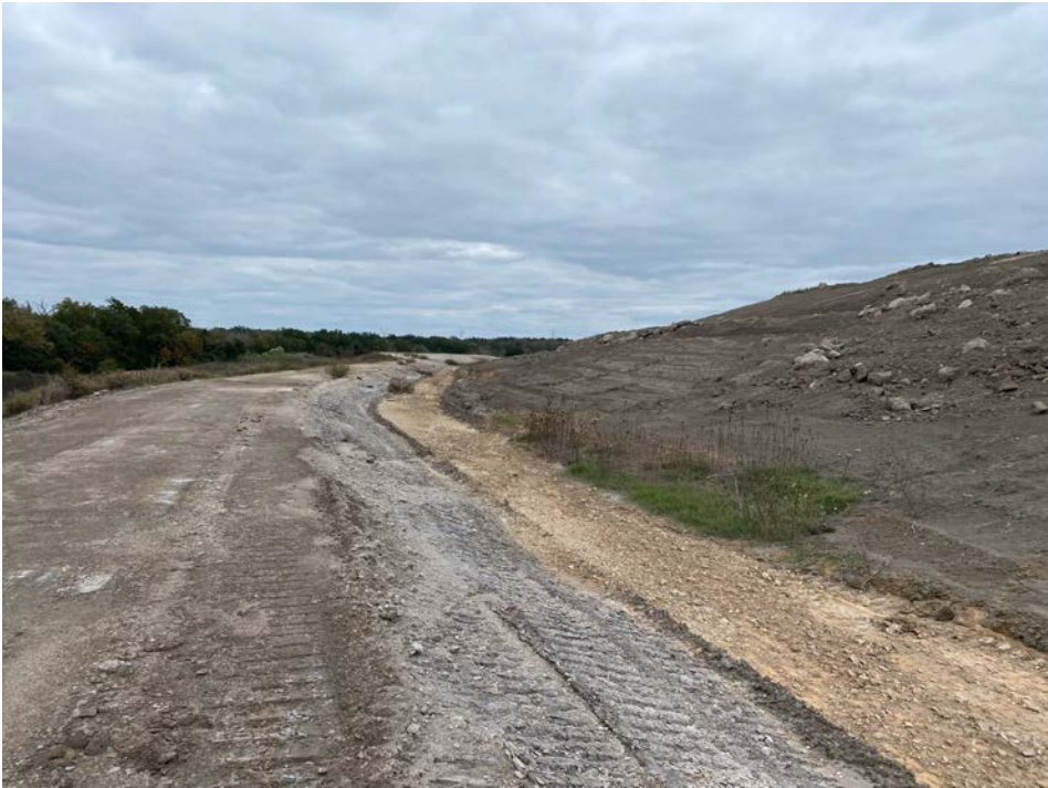
Photo No. 5 – North perimeter ditch, view northeast.
