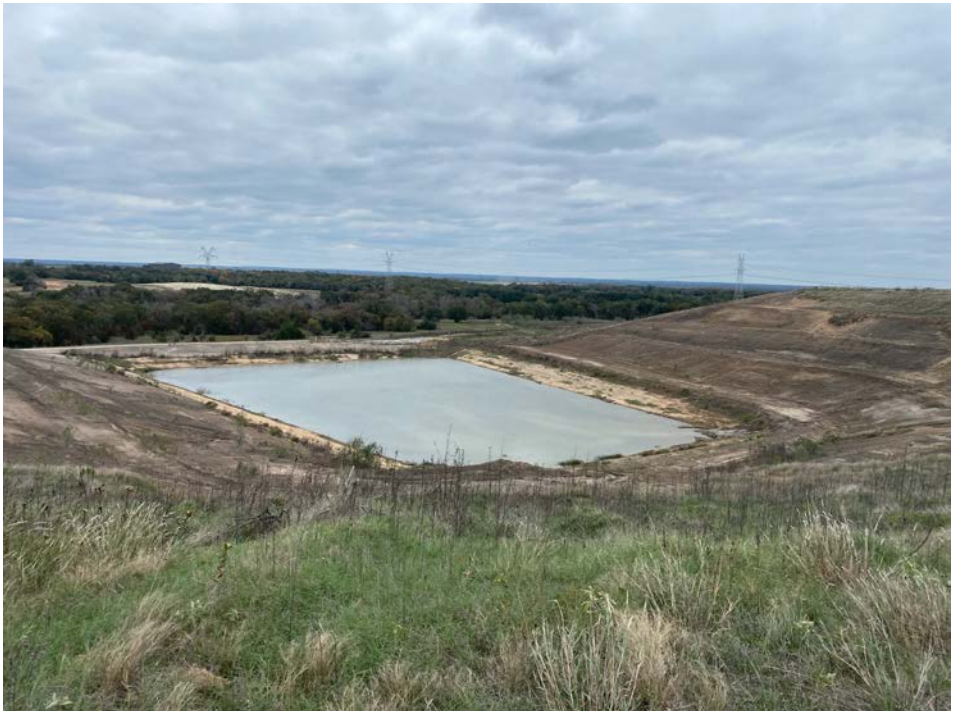
Photo No. 14 – Stormwater Pond 003, view southeast
